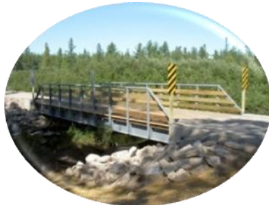
Schoolcraft Co. Snowmobile Assoc. Sturgeon Hole Creek 50 Ton, 40' Span
