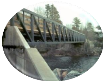
Hiawatha Trails Inc. Escanaba River H15, 125' Span
